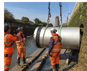
Installation of WaStop non-return chamber in Stratford, East London
